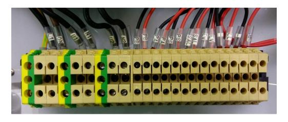
ELECTRONIC BUSBAR CONNECTION FOR 230V AC POWER SUPPLY FIG. 4-4
