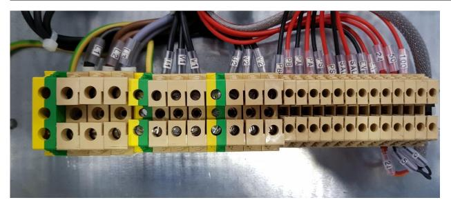
ELECTRONIC BUSBAR CONNECTION FOR 380V AC POWER SUPPLY FIG. 4-5
