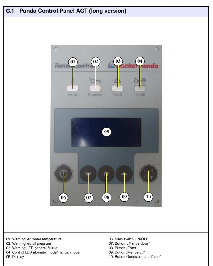
Fig. G.1-1: Front Panda Control Panel (long version)
