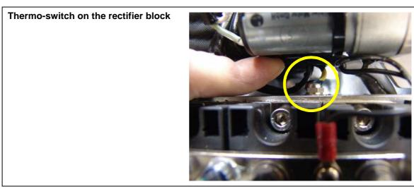
Fig. A.3.7-7: Thermo-switch on the rectifier block
