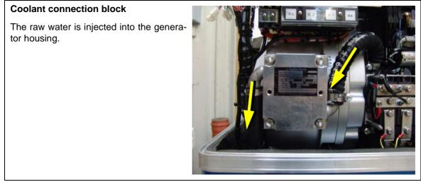
Fig. A.3.2-5: Coolant connection block
