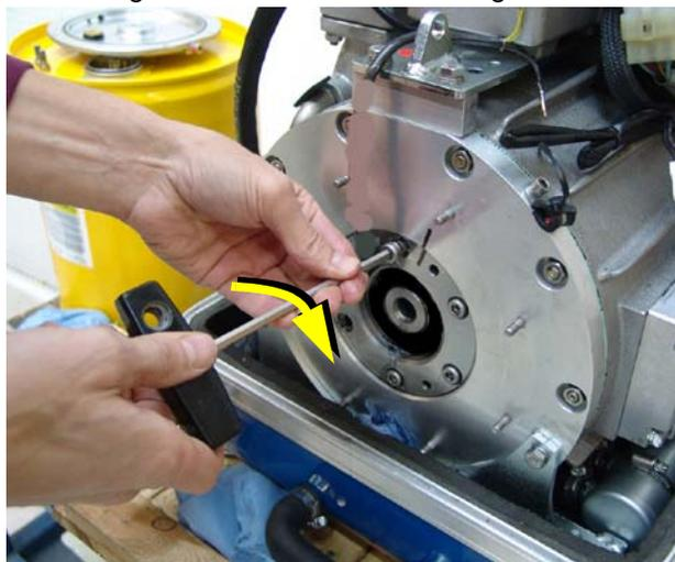
Screw in thread rod into the thread hole of the generator shaft as far as possible.
