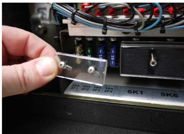
3. Using the fuse extraction tool, remove the fuse and replace it with a new one.
