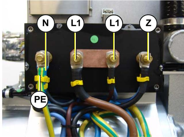
Fig. 8.5.0-2: Wiring diagram HP1 - 230 V / 50 Hz
