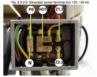
Z1.1 H1.1 **Z**1 Z1.2 H1.2 H2.2 Z2.2 **H2 Z2** H2.1 Z2.1 3 Neutral Ground 120V/60Hz Neutral Hot Hot Ground 230V/60Hz
