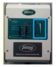
Figure 3: DDC box with load indication
