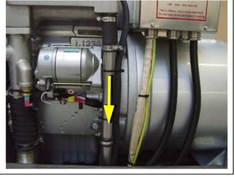
Fig. A.3.3-3: Freshwater backflow
