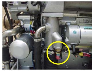
Fig. A.3.7-3: Thermo-switch at exhaust connection
