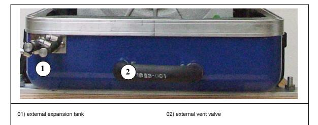
Fig. A.2-2: Generator Connections
