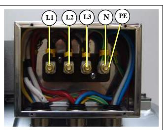
Fig. A.3.6-9: Generator Power Terminal Box 400V/50Hz
