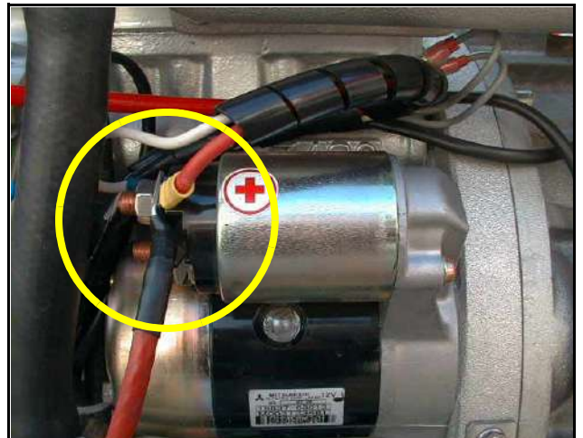
Fig. 6.10.1-1: Positive Battery Cable
