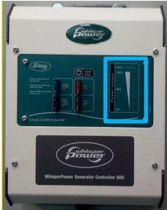
Figure 3: DDC box with load indication
